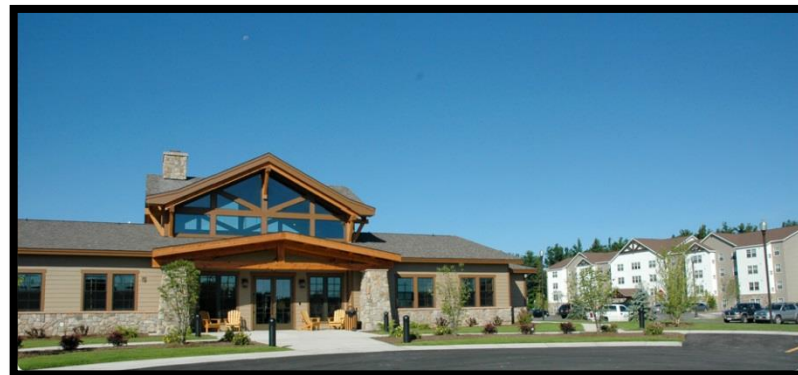
Fort Drum's Privatized Unaccompanied Housing, The Timbers
